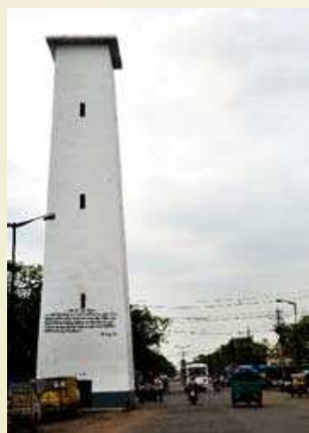
Trigonometric Survey tower on B.T. Road, Kolkata. The inscription says, “G.T.S. Tower. This 75-ft brick tower was built in 1831 for the Great Trigonometric Survey conducted by George Everest, Superintendent of Great Trigonometric Survey and Surveyor General in charge of all topographical & revenue surveys.”
