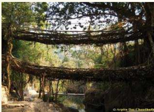
Double-decker root-bridge of Umshiang formed by Ficus elastica roots
