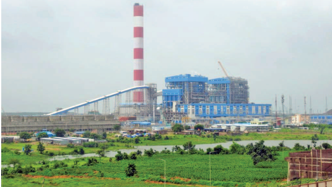
Ultra-Super Critical Thermal Power Plant at Khargone
