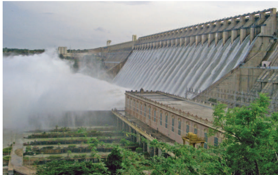
Nagarjuna Sagar Dam. Photo: WikiCommons
