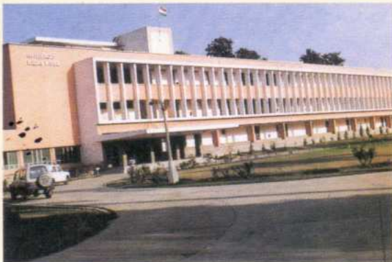
A facade of Central Road Research Institute, New Delhi
