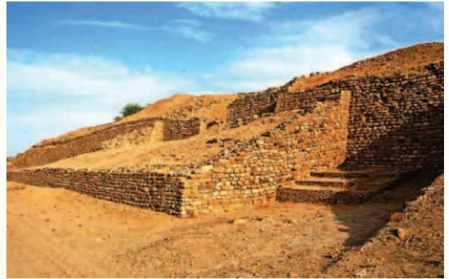
The remains of the magnificent Northern wall of Dholavira that is believed to have been built as a protection against storm surges and tsunamis.
