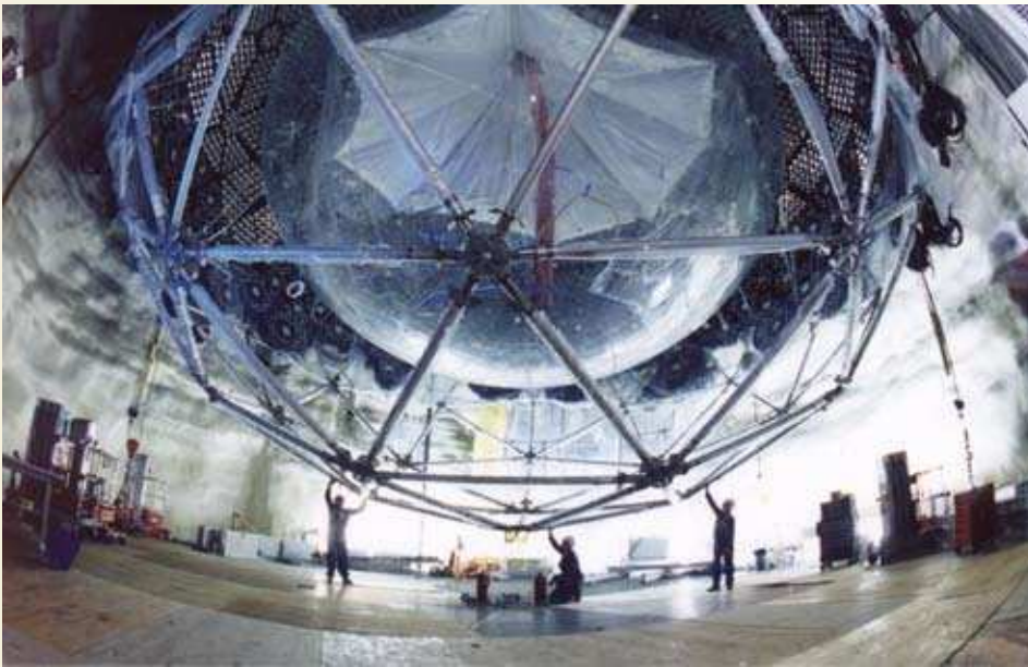
The Sudbury Neutrino Observatory in Canada is a scientific masterpiece (here seen during construction). Designed to detect solar neutrinos, it is a spherical tank measuring 12.2 metres in diameter and is located 2 kilometres beneath the Earth's surface. It is filled with heavy water.
