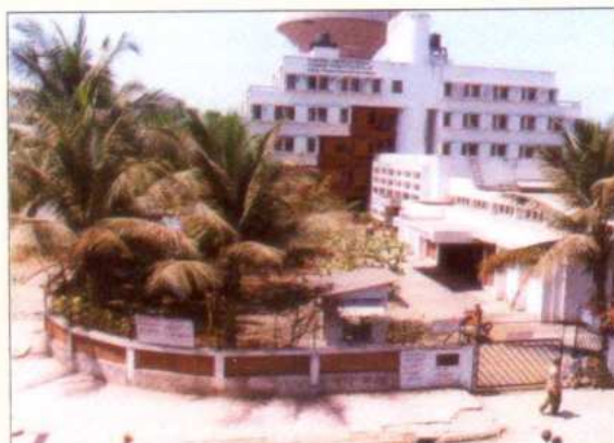
IWSA Building Complex at Vashi
