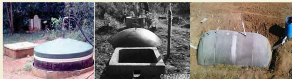
KVIC biogas plant (left) Deenbandhu biogas plant (centre) Balloon biogas plant (right)
