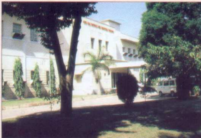
Shriram Institute for industrial Research on University Road, Delhi
