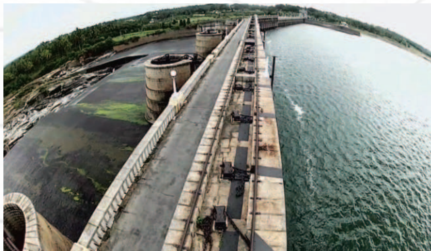
Bird's eye view of the Krishnaraja Sagar dam. (Photo: Matiur Rahman)
