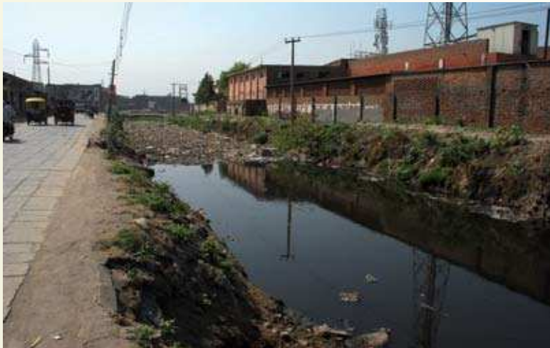
Waste in a large drain such as this finally flows into the Yamuna River. Unless drains are diverted and only treated waste water let into the river no river cleaning project can succeed.
