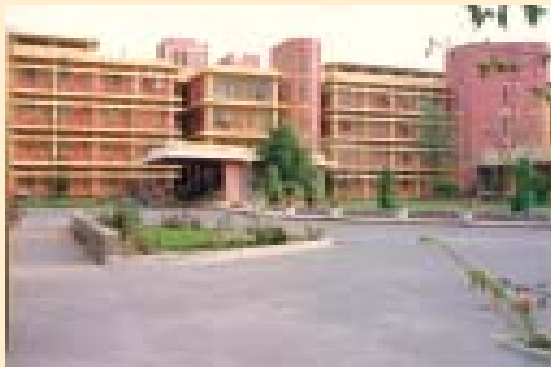
Nuclear Research Laboratory building in the I.A.R.I. campus, New Delhi
