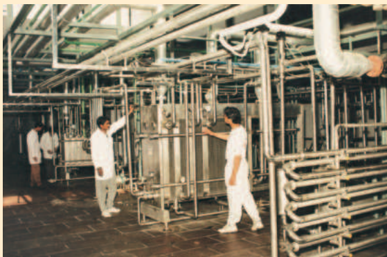
Inside view of the Model Dairy Plant
